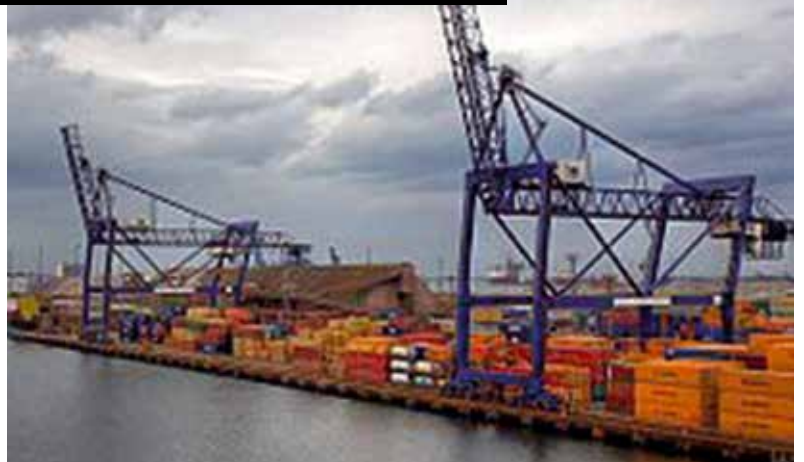
container terminal, Teesport
